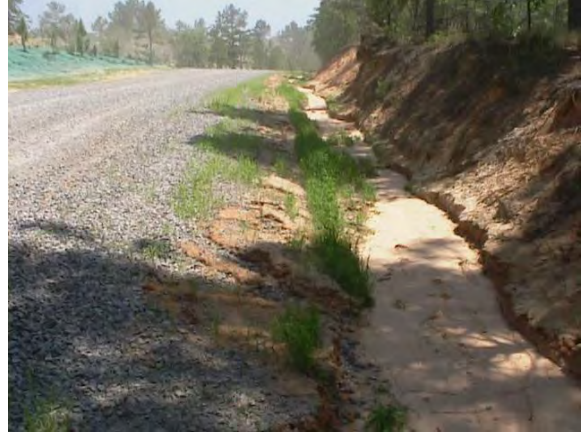
Figure C-18. McKellers Road – Adequate checkdams and in-time repairs would have prevented a complete washout.
