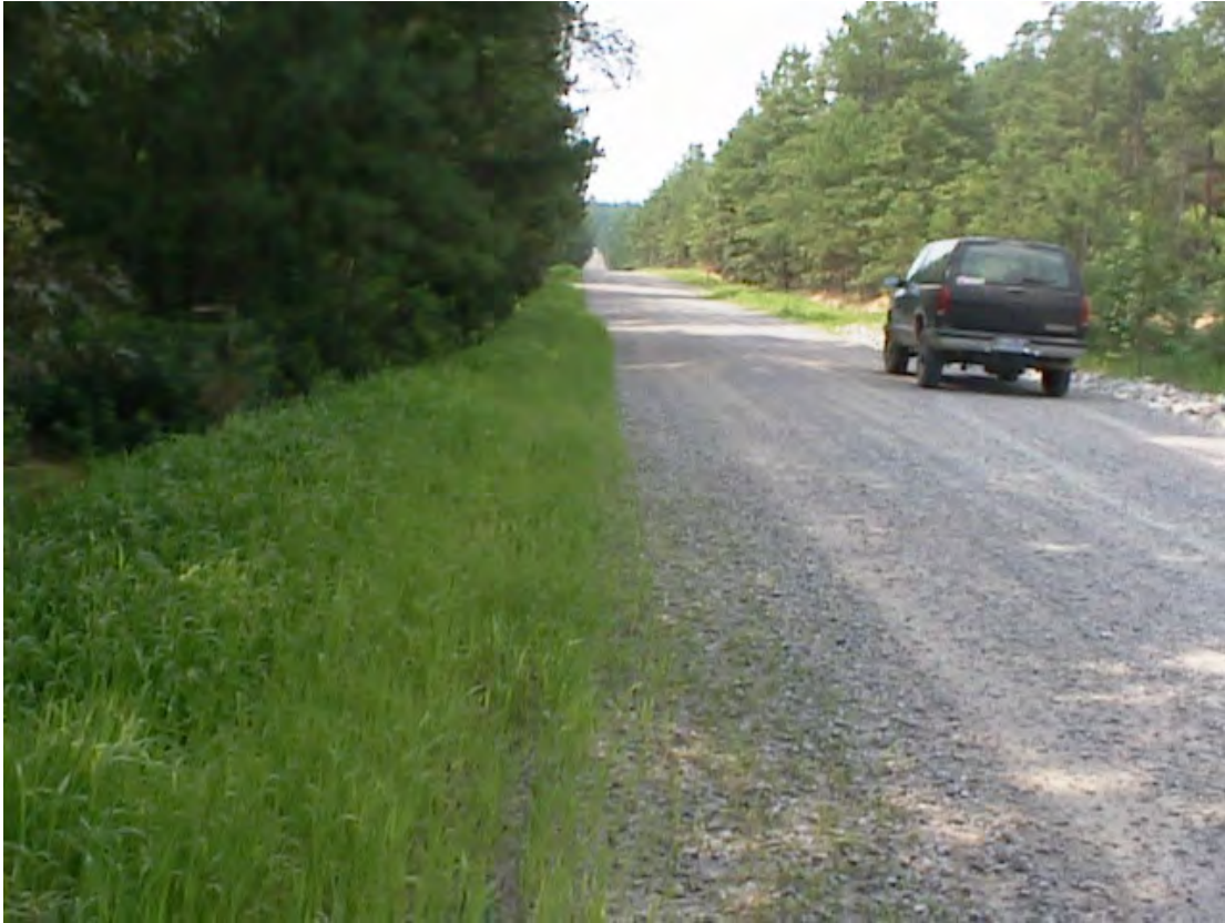
Figure C-17. Revegetated 2-mile section of McKellers Road.
