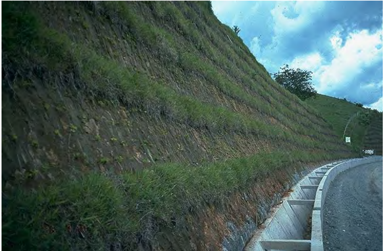
Figure B-2. Hedge grasses may be the only choice of vegetation on steep slopes.
