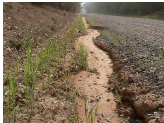
Figure F-10. Vegetative control measures are not a cure-all for all erosion problems, e.g., Fort Bragg gully erosion (left) and McKellers Road erosion, Fort Bragg (right).
