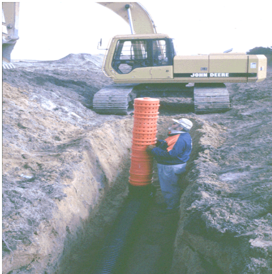
Figure C-6. Higginbottom riser installation at Normandy DZ, Fort Bragg, NC.
