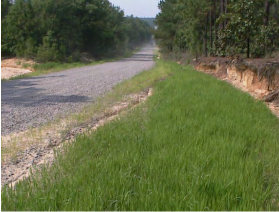
Figure C-18. McKellers Road – Adequate checkdams and in-time repairs would have prevented a complete washout.
